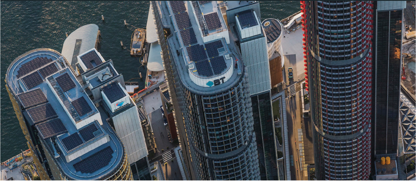
International Towers, Barangaroo, part of the Climate Positive Precinct. Photo courtesy of Barangaroo Delivery Authority
